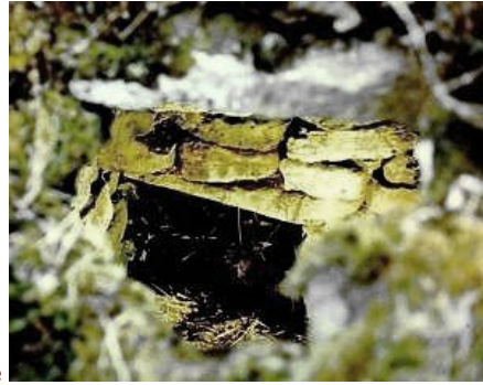
Sweathouse doorway seen through a hole in the corbelled roof, Cultia, county Leitrim
