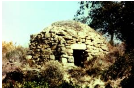
Corbelled shepherd-hut, Artajona (Navarra), Spain and a gariota or casela in Quercy, France.
